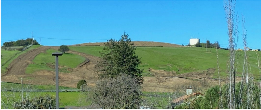
Figure 7: Oat Hill Grading In Progress
