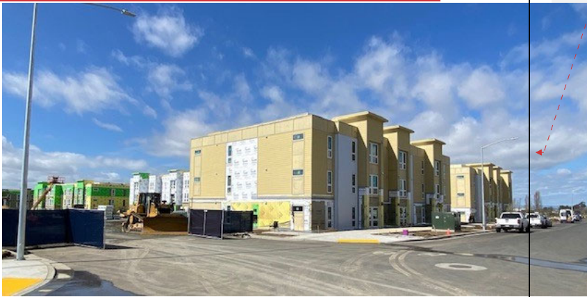
Figure 1: Lemos Point Modular Apartments Under Construction
