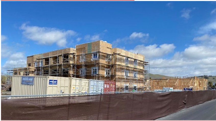
Figure 4: Napa Cove Apartments Construction
