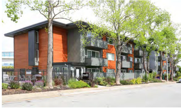
Three21 @ Belmont Apartments located at 321 Oxford Way
