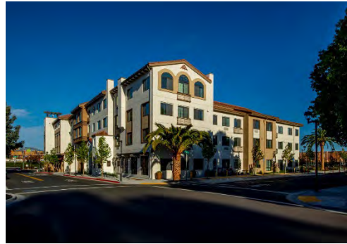
Firehouse Square 1 located at 1300 El Camino Real
