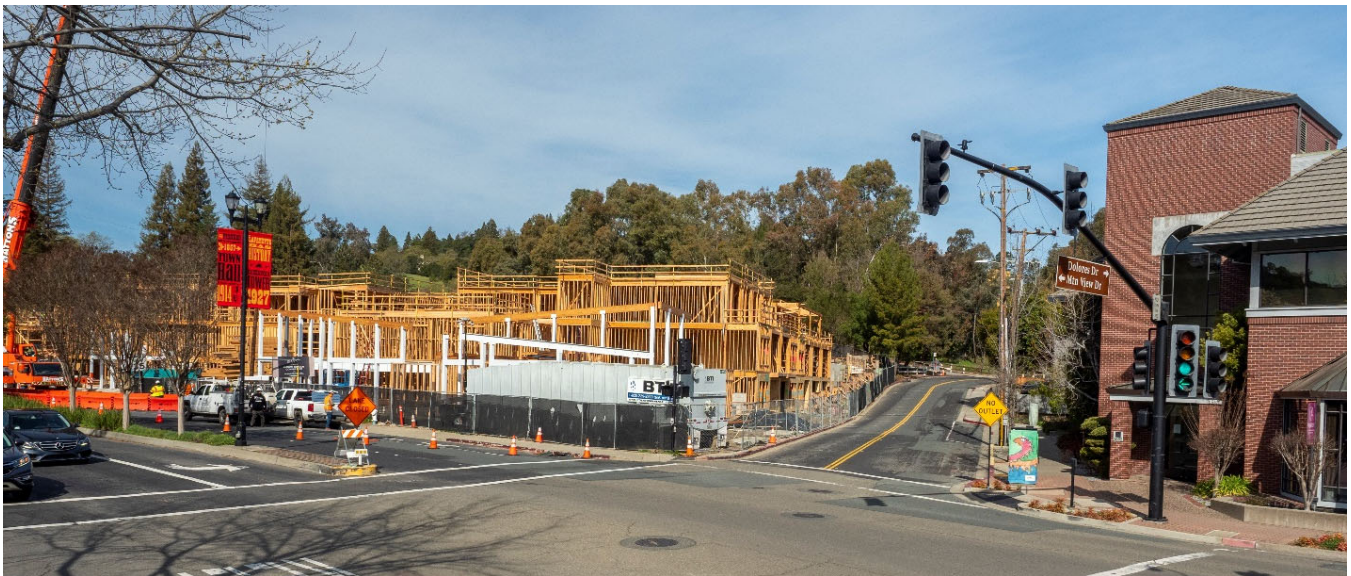
The Brant under construction in 2022.
