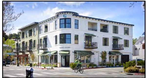
G Square Living is a market-rate, mixed-use development in San Rafael, CA. It has 10 units with a density of 59 dwelling units per acre.
