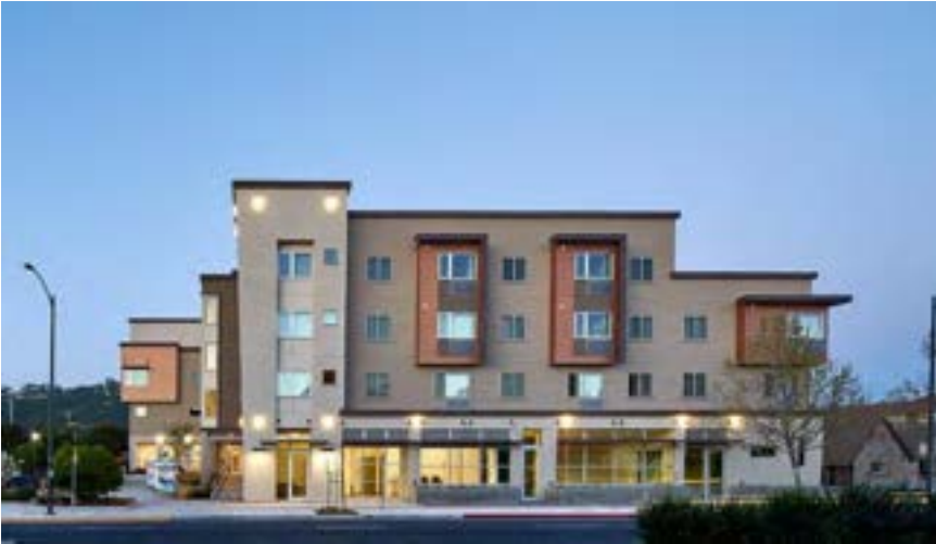
Existing Building Elevation
