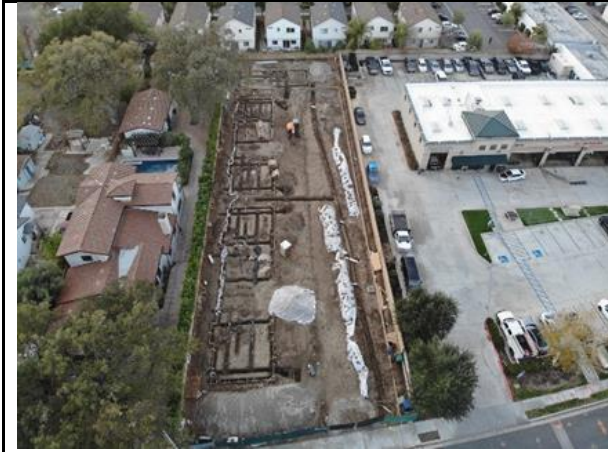
Existing: Looking West
