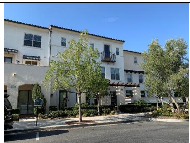
Existing: Looking West
