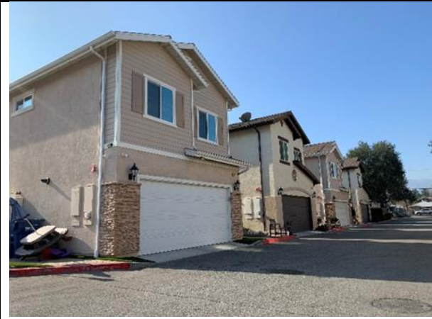
Existing: Looking Southwest
