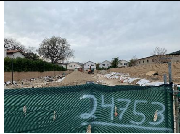
Existing: Looking West
